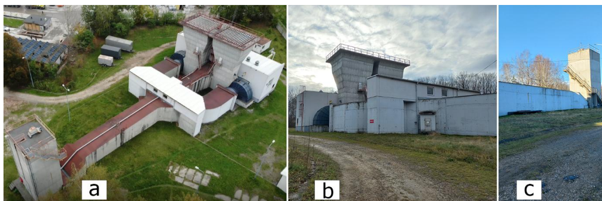
135 Figure 1: Views of the monitored ventilation shaft, including the main channel and fan station with two diffusers.
