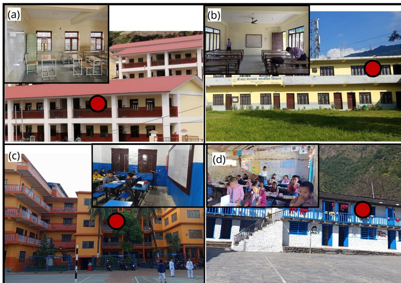
Figure 7: Example of school buildings and classrooms associated with different risk levels. (a): low risk levels with earthquake-resistant buildings. (b): medium risk level with the RCC building, (c): high risk levels with the RCC building, (d): very highrisk levels with the traditional stone and mud building. The black-contoured red circle represents the location of the inset classroom images for each school building.
