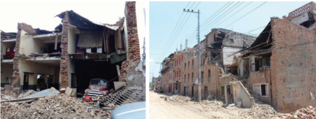
Figure 3. Fallen bricks near building from front wall collapse (left) and partial wall collapses (right), 2015 Gorkha Nepal earthquake (Credits: Anne Sanquini, (left), Bipin Shrestha (right), provided by Earthquake Engineering Research Institute)
