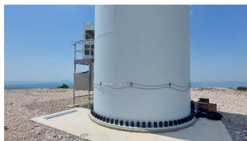
Figure 2a. Rogowski-coil current sensors at the WT4 tower
