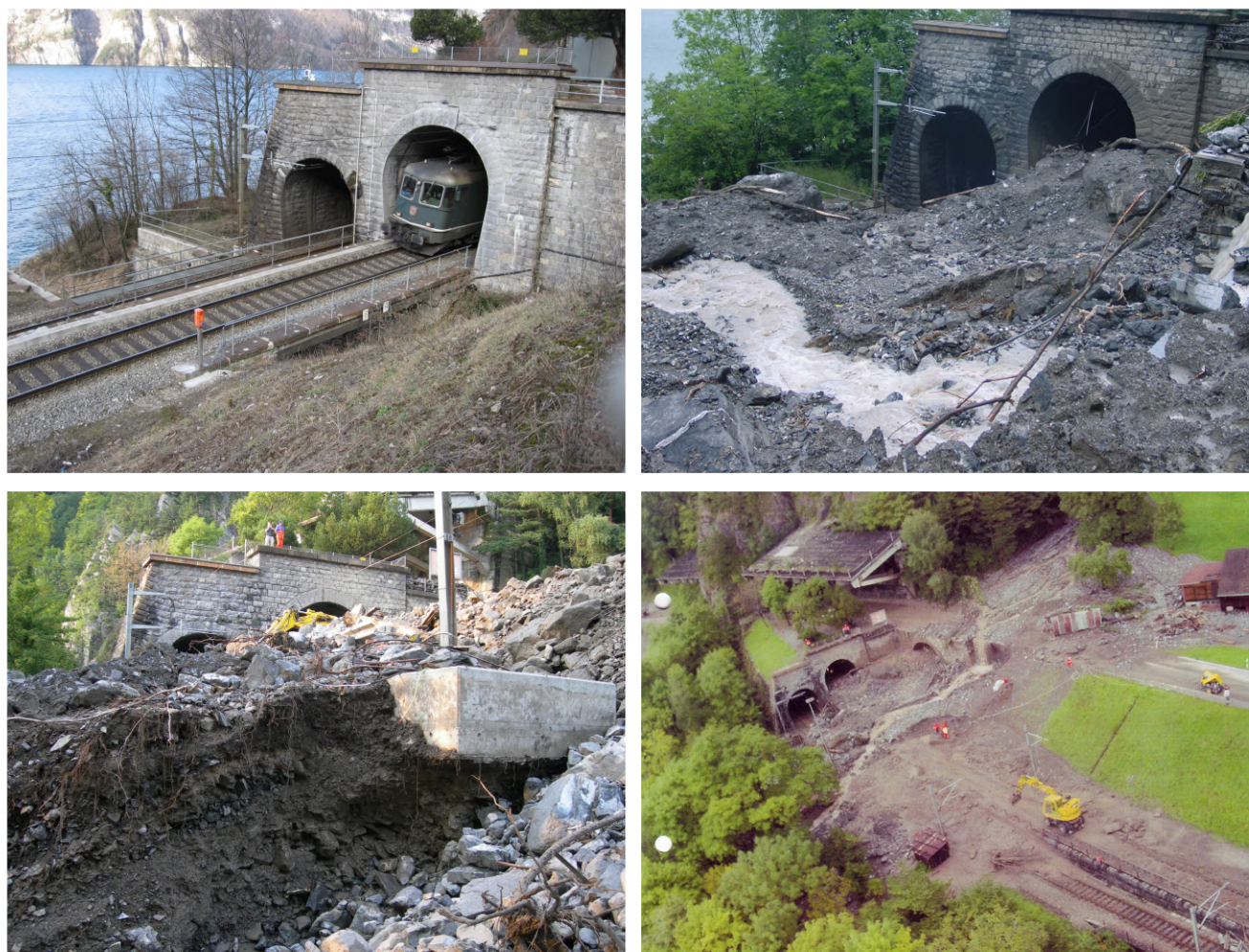
Figure B1. Illustrations from the Dornibach railway crossing in Canton Uri, Switzerland. Upper left is before the event. Other illustrations show the railway infrastructure after the event of August 24th, 2005.
