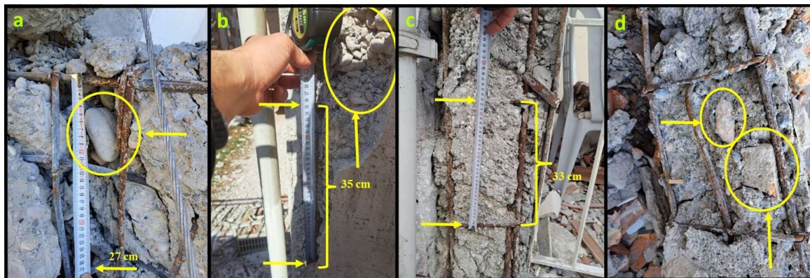
Figure 7. Reinforcement detailing deficiencies and material-quality-related damage observed in older RC buildings following the February 6, 2023, Kahramanmaraş earthquake sequence.
