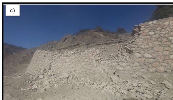
Figure 15. Damage observed in gravity-type stone retaining walls
