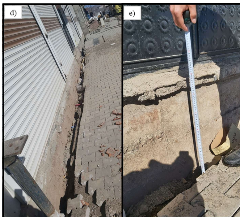
Figure 11. Settlements of superstructure induced by bearing capacity loss and differential foundation settlement
