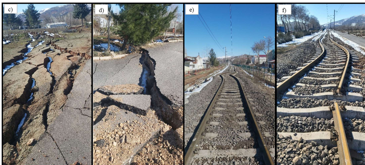
Figure 13. Lateral spreading observed in the ground
