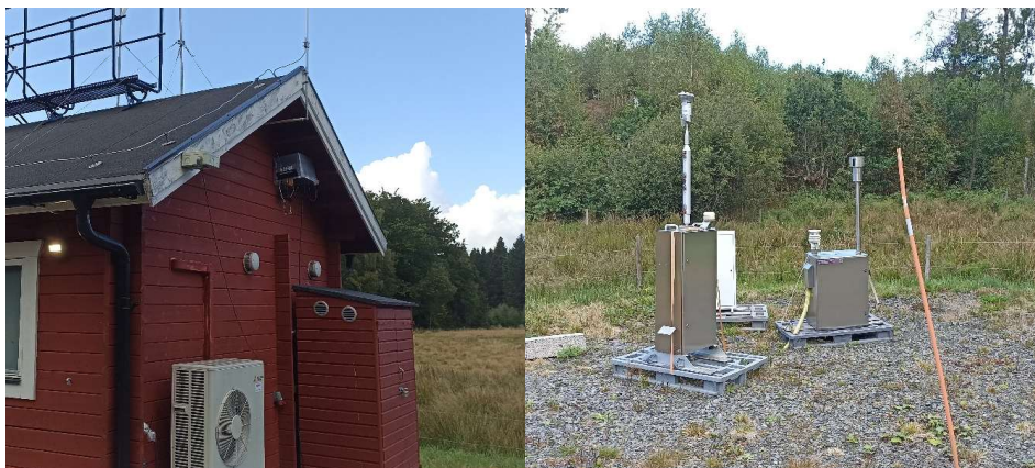
Figure H1: Installation of SPS30 and SEN55 sensors (left) and a Palas Fidas (right) at Hyltemossa monitoring site.
