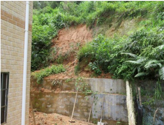
93 Figure 2: Photos of the on-site investigation of shallow landslides.
