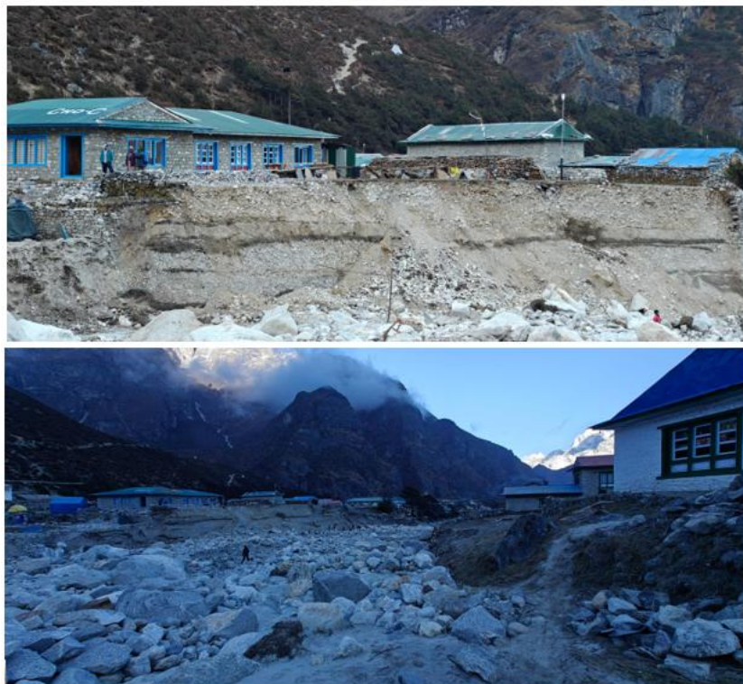
Figure S10 Ongoing channel erosion and debris deposition along the Thame stream in Thame Valley, Nepal, showing the close interaction between active geomorphic processes and nearby settlements and infrastructure. Photo by N. Khadka, 2024.
