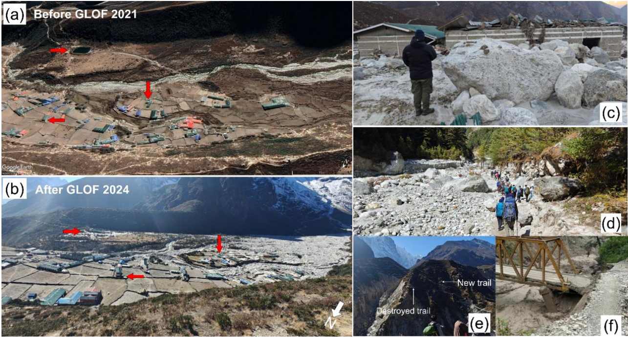
398 399 Figure 10: Impacts of Thame Valley GLOF. Thame Valley (a) before and (b) after GLOF, (c) the damaged Thame school, 400 walking trails (d and e) and the motorable bridge (f). The red arrows show common feature/buildings on panels (a) and (b).
