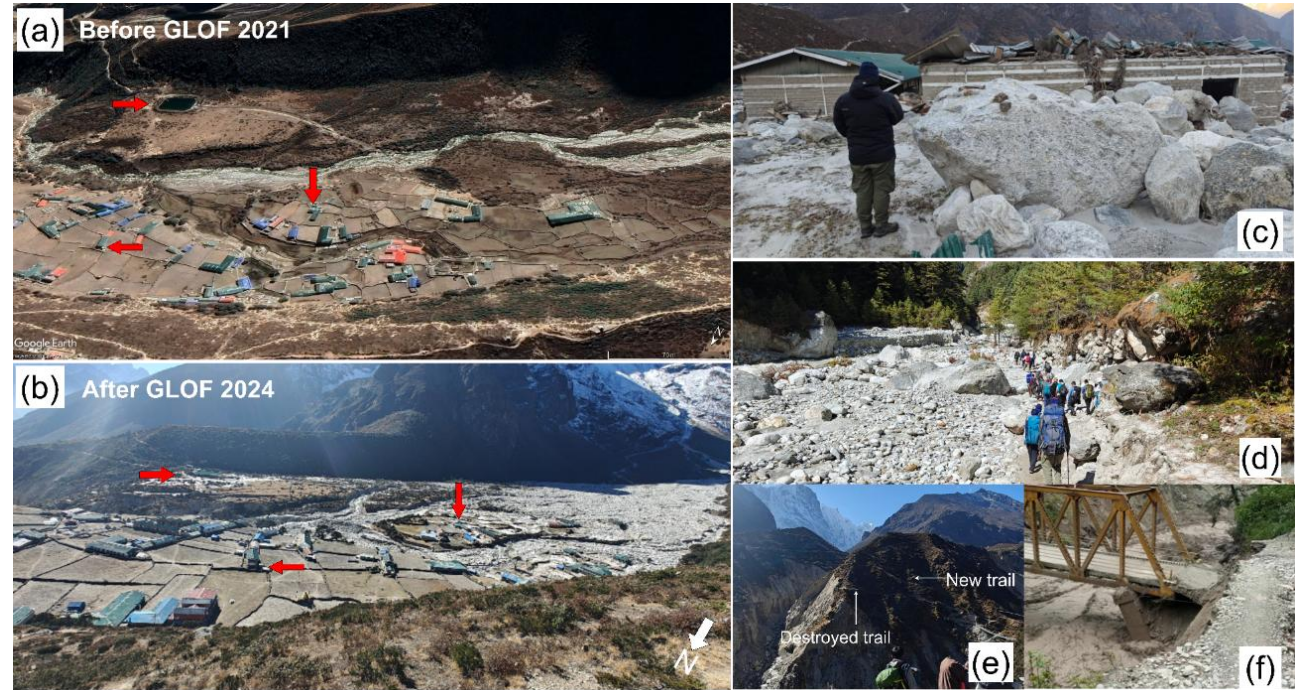
Figure 10: Impacts of Thame Valley GLOF. Thame Valley (a) before and (b) after GLOF, (c) the damaged Thame school, walking trails (d and e) and the motorable bridge (f). The red arrows show common feature/buildings on panels (a) and (b). Source: The picture (a) is sourced from © Google Earth 2024; images: © CNES/Airbus, Maxar Technologies, Airbus whereas others from Field Study, 2024.
