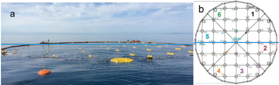
456 Figure 1. Large ring in fold-up form at sea, during deployment just prior to finish the opening of air- 457 valves. The front part of the large steel-pipe ring is already underwater. Almost all top-buoys of the 45 458 small-ring-compacted mooring lines are visible. In the front still outside the ring, the yellow drag 459 parachute and orange pick-up buoy are floating. (b) Location named "Temp Array" (orange dot) off 460 southern France. The mooring is well east of main neutrino telescope 'NT' site "ORCA" of KM3NeT 461 (Adrián-Martinez et al., 2016) and just northeast of the former ANTARES NT-site. Isobaths are given 462 every 100 m. (c) Layout of the large-ring mooring viewed from above, with steel-cable grid and small-
