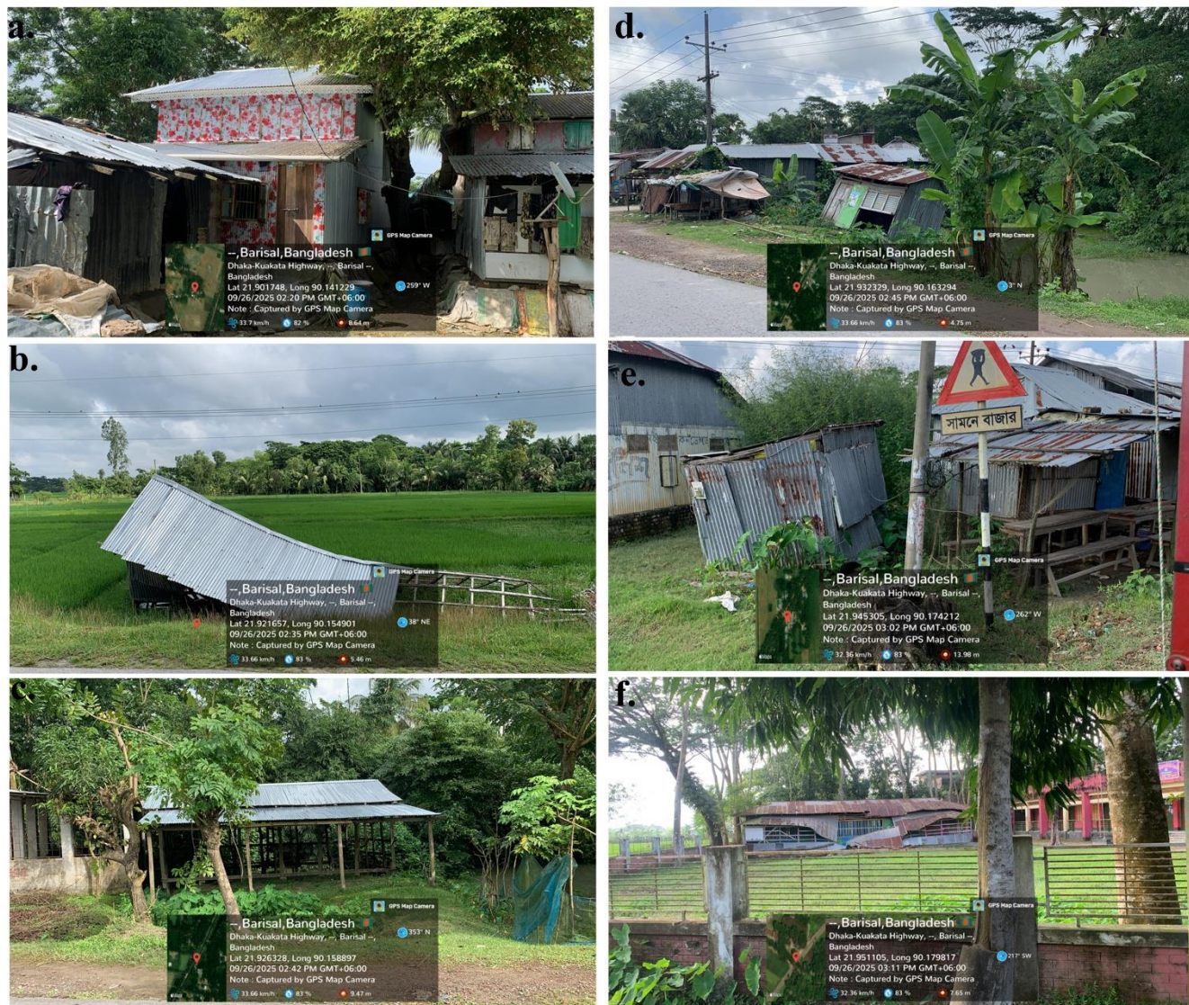
Figure 6 Damages of Cyclone Remal (2024) found during field validation in Kala Para Subdistrict.
