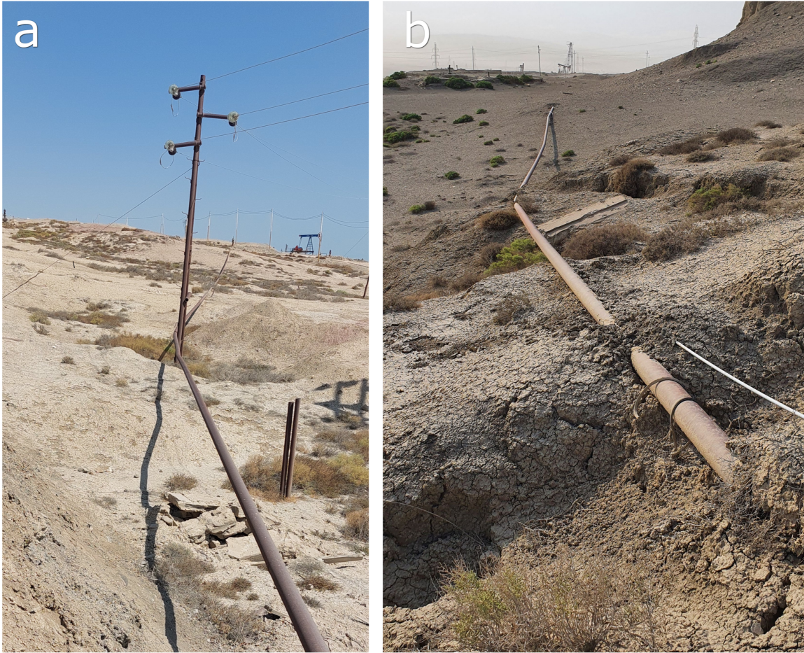
Figure 5: Example of infrastructures built across the creeping mud flow at Lokbatan MV. (a-b) ongoing flow movement causes deformation of the pipeline.
