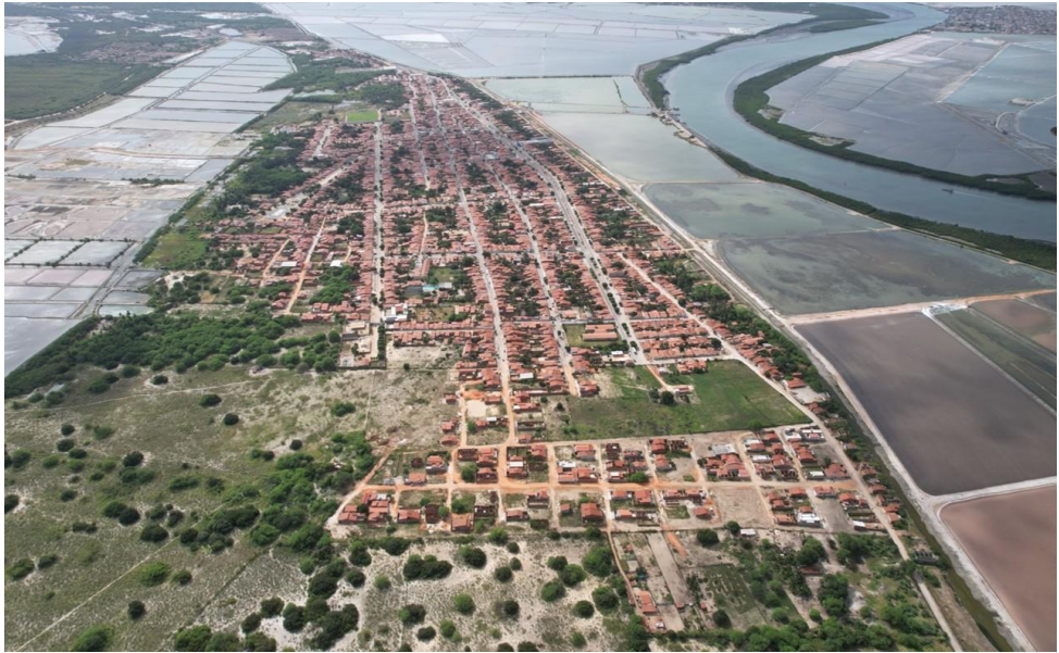
Figure 8: Aerial image of downtown Grossos, showing the dikes that control the levels of salt flats on the outskirts of the urban area. Photograph by the study authors. © Authors, 2026.
