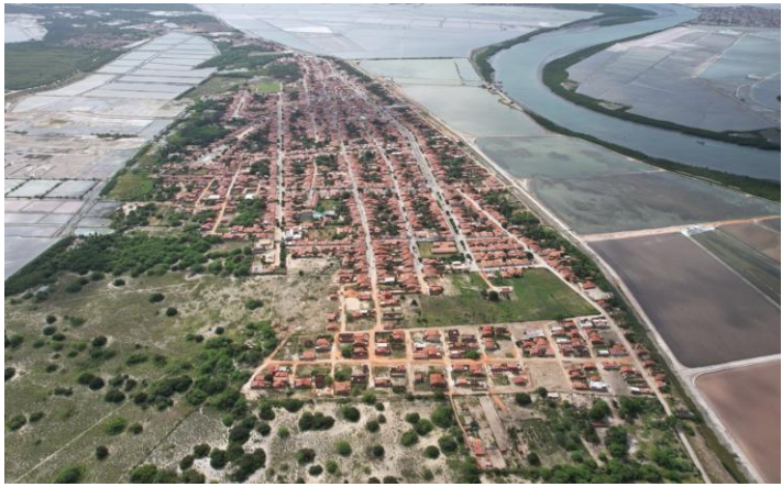
Figure 8: Aerial image of downtown Grossos, showing the dikes that control the levels of salt flats on the outskirts of the urban area. Photograph by the study authors. © Authors, 2026.
