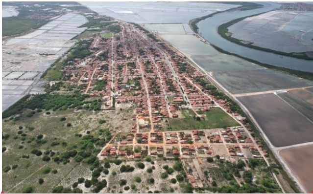
Figure 27: Flood relations. A—Aerial image of downtown Grossos, showing the dikes that control the levels of salt flats on the outskirts of the urban area. B—News report on a collapsed dike in Grossos in 2024. Panel A photograph by the authors (2025). Panel B adapted from Mossoróhoje (2024). © Mossoróhoje.
