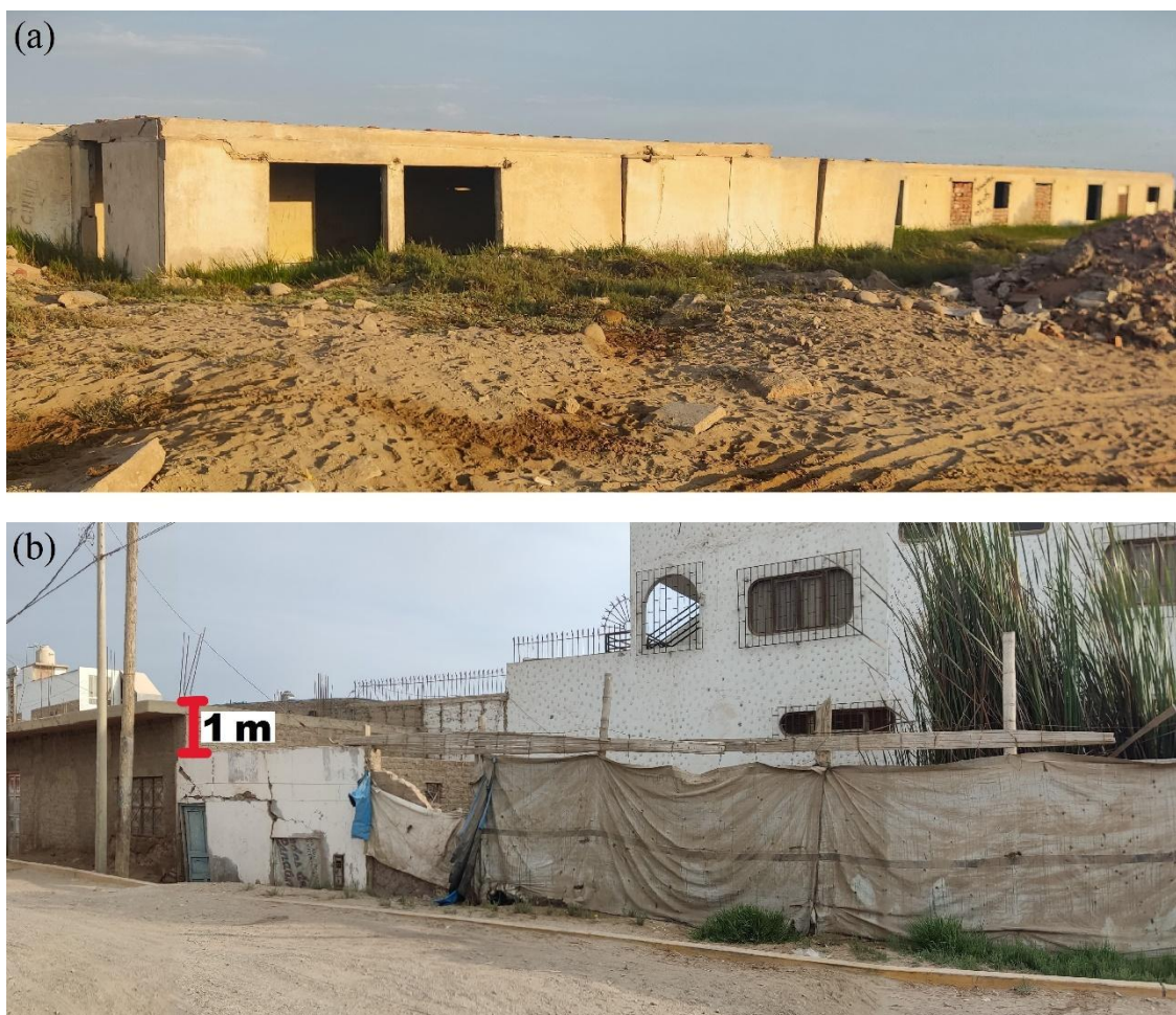
Figure 2: Houses affected by soil liquefaction during the 2007 Pisco earthquake: a) Abandoned house, showing settlement with 30 cm of subsidence; located along the extension of Av. Manuel Pardo, near the Pisco Playa – Boca de Río sector, adjacent to wetland H-01. Subsidence of 1 m with walls exhibiting variable inclination. b) Settled house with 1 m of subsidence and forward tilting, now uninhabitable, where totora (bulrush) has grown; located on Alfonso Ugarte Street, Pisco Playa Sur, within the extended area of wetland H-01. (Baez et al., 2023)
