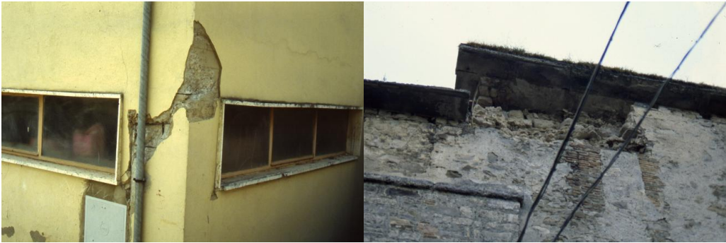
Figure 2. Example of damage caused by the 1990 event in the village of Pietragalla (left) and Cancellara (right). Intensity 7 and 6-7 MCS from Tertulliani et al., (1992), respectively.
