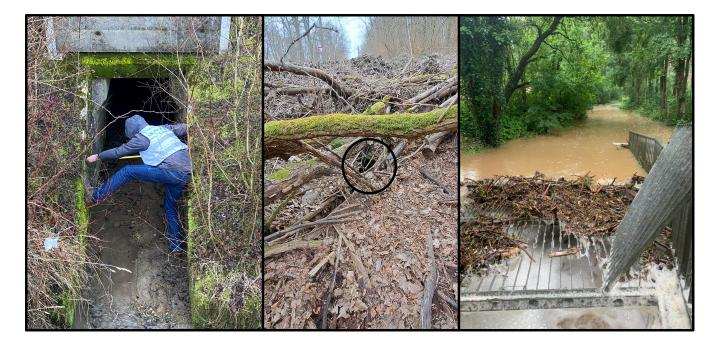
**Figure 4.** left: inspection of an unsurveyed culvert with slight sedimentation, middle: extreme logiam in front of an unsurveyed culvert (see black circle for culvert location), right: blocked culvert during the flood event at 9th of July, 2021 (Feuerwehr Reichenberg (2021b), https://ff-reichenberg.de/einsatzberichte/1752-hochwasser-strasse-ueberflutet/)
