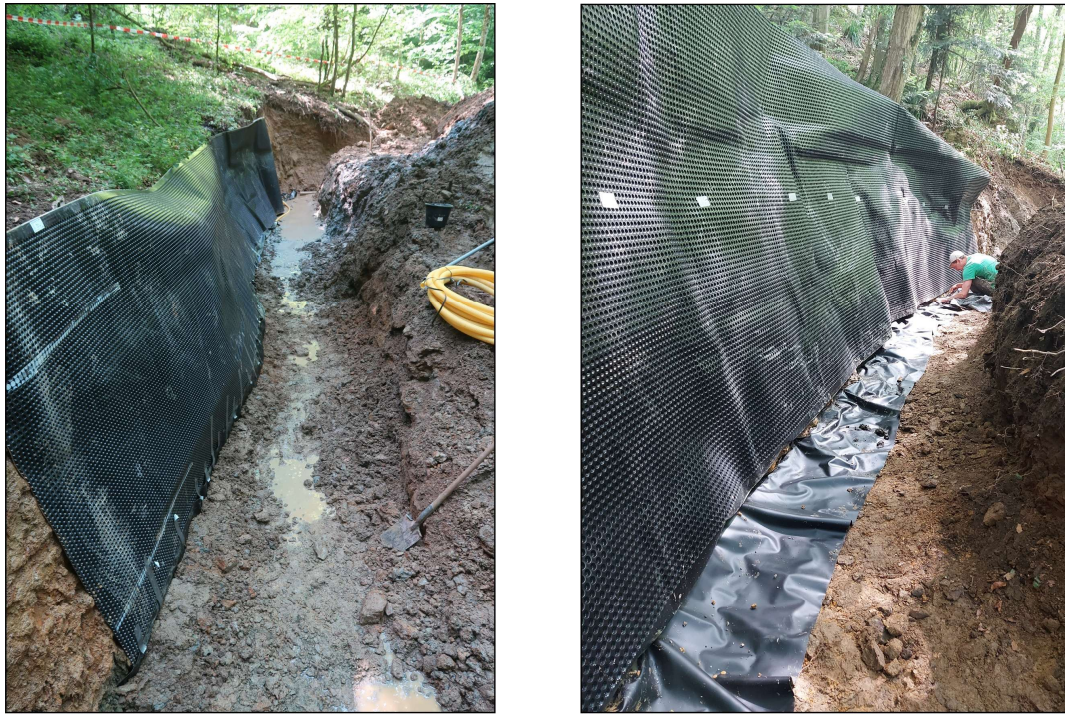
Figure A1. Trenches during construction
