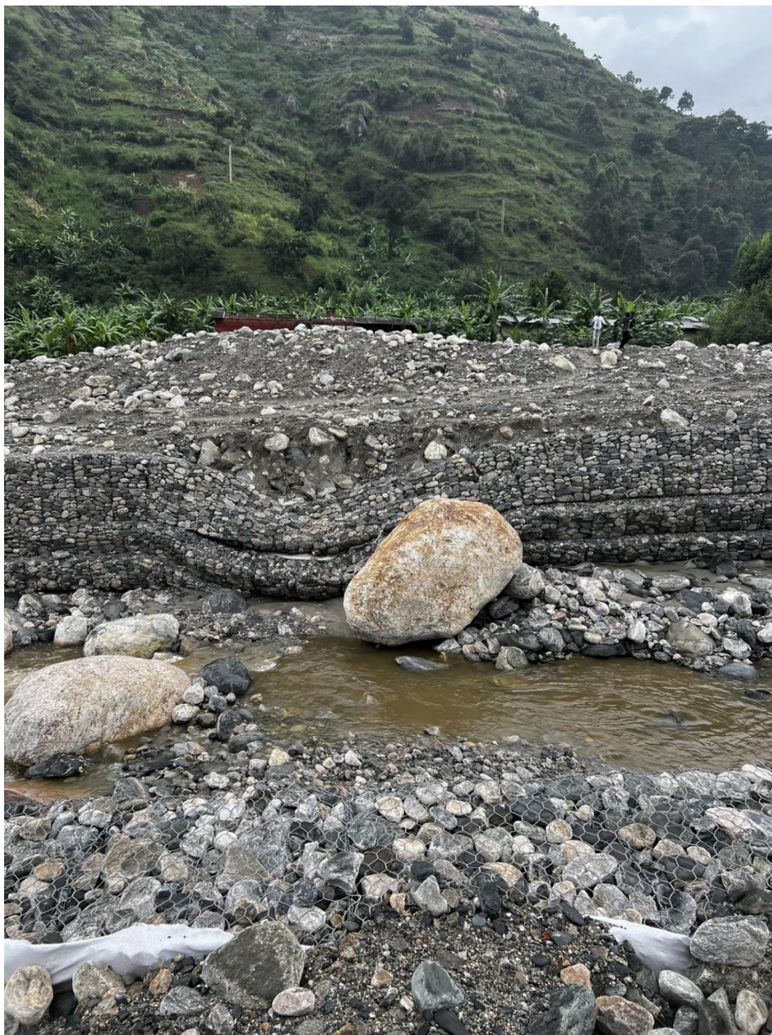
Figure H2: 0.21387N, 30.00558E, 7 June 2023 (damaged gabions).
