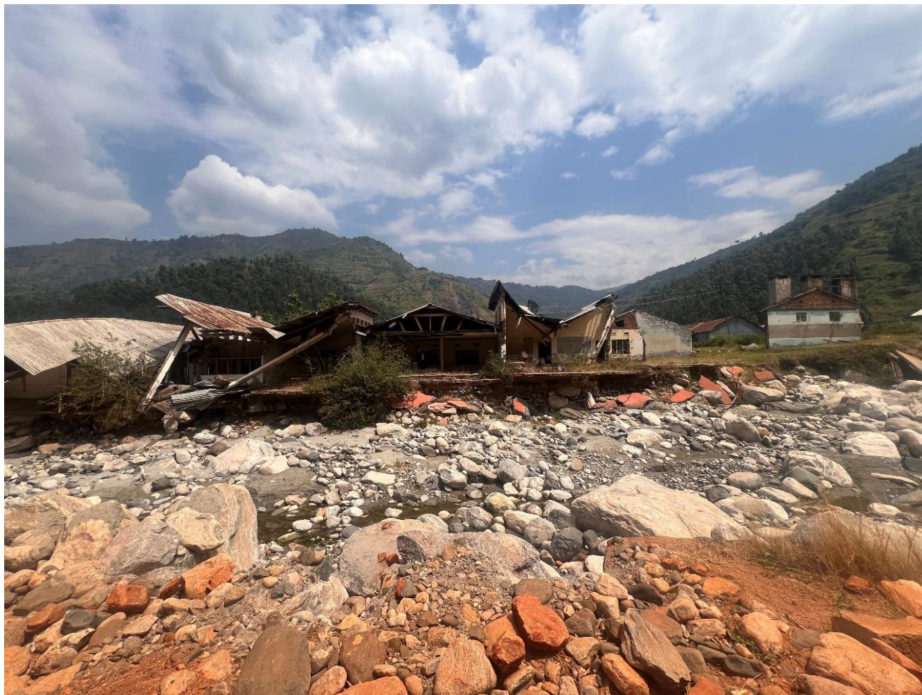
Figure F2: River cliff style erosion of house foundations in Kilembe, 0.20603N, 30.00822E – 24 July 2024.
