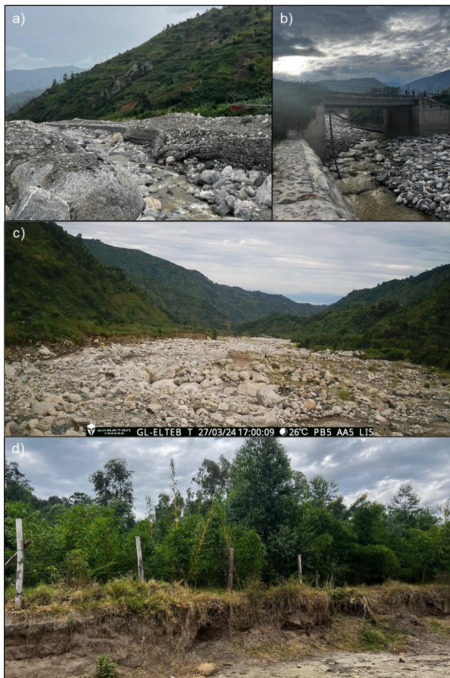
815 Figure L1 – Photographs taken during June 2023 field reconnaissance: a) collapsed gabions adjacent to Kilembe town (for scale: 8 m channel width); b) channelisation using concrete embankments in Kilembe town centre (10 m channel width under bridge); c) photo from a camera transmitting photos at 1-minute intervals 5 km upstream of Kilembe town centre for flood early warning; d) river bank stabilisation adjacent to Kasese town including asper bamboo (4 m fencepost spacing).
