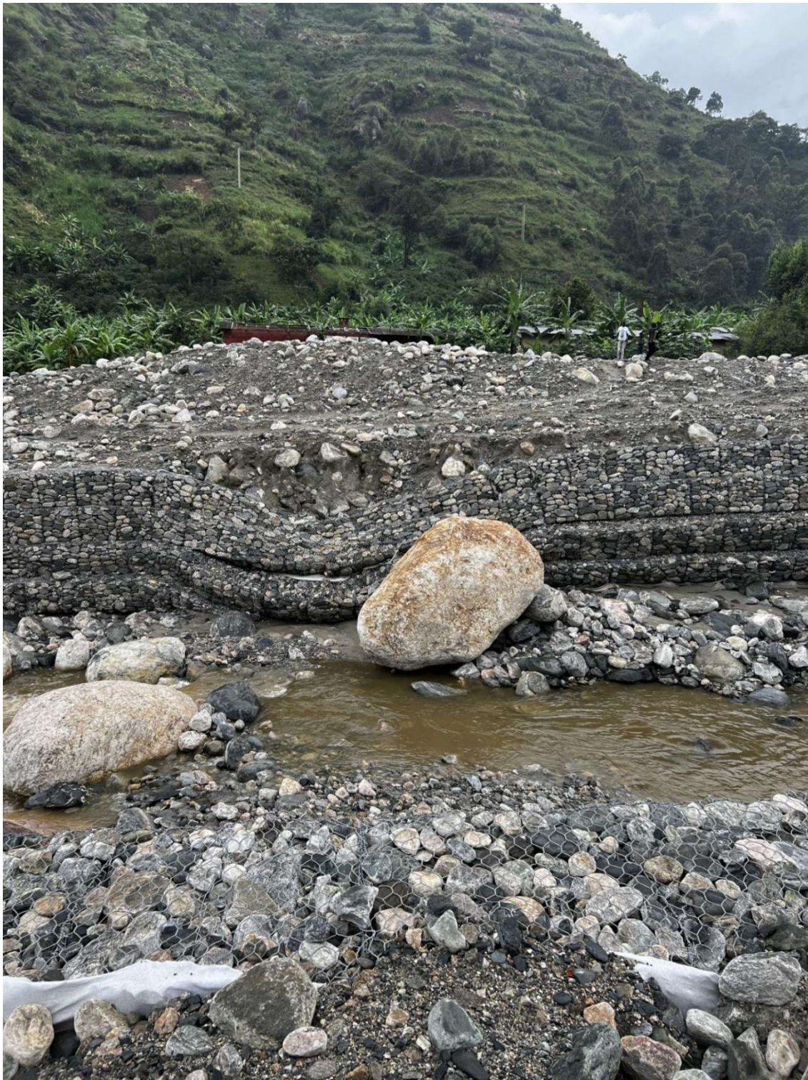
Figure H2: 0.21387N, 30.00558E, 7 June 2023 (damaged gabions).
