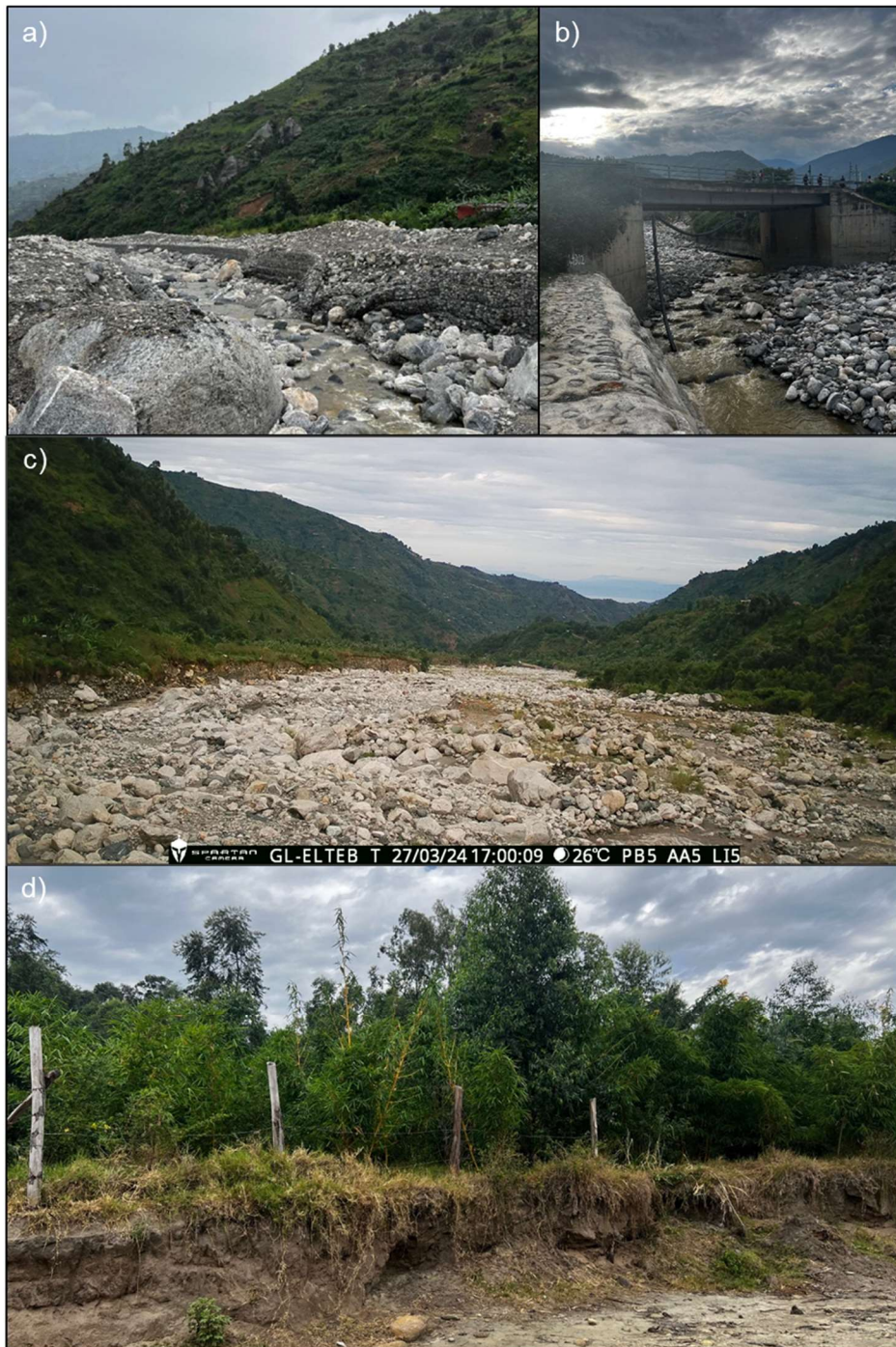
Figure M1 – Photographs taken during June 2023 field reconnaissance: a) collapsed gabions adjacent to Kilembe town (for scale: 8 m channel width); b) channelisation using concrete embankments in Kilembe town centre (10 m channel width under bridge); c) photo from a camera transmitting photos at 1-minute intervals 5 km upstream of Kilembe town centre for flood early warning; d) riverbank stabilisation adjacent to Kasese town including asper bamboo (4 m fencepost spacing).
