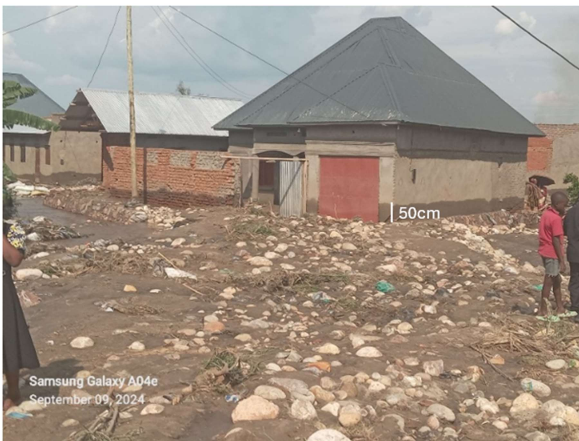
942 943 Figure L1: Photograph following flooding in Kasese town evidencing the inundation level and post-flood ground 944 contamination. Photograph provided by the Ministry of Water and Environment.
