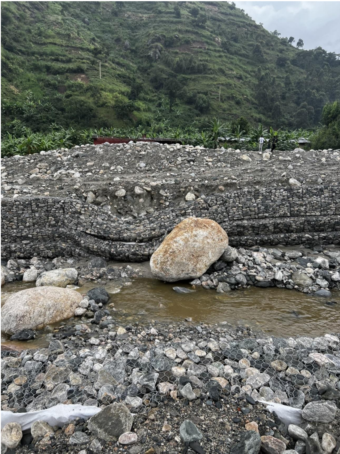
Figure H2: 0.21387N, 30.00558E, 7 June 2023 (damaged gabions).
