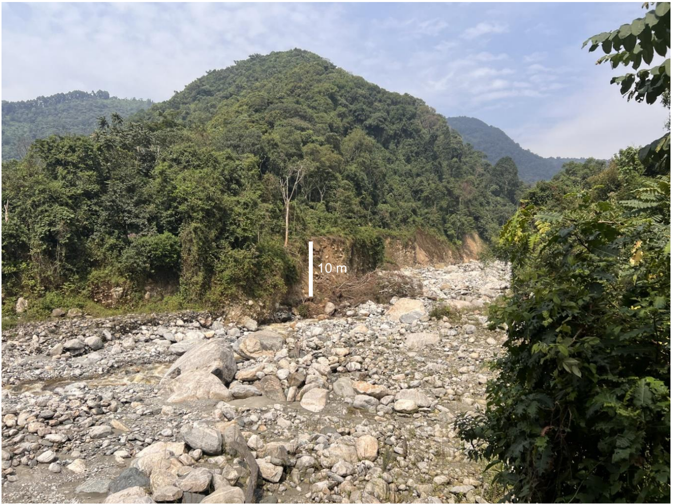
912 913 Figure I2: Landslide scar at 0.23758N, 29.97570E – 1 August 2024. 914 915 916 917 918 919 920 921 922
