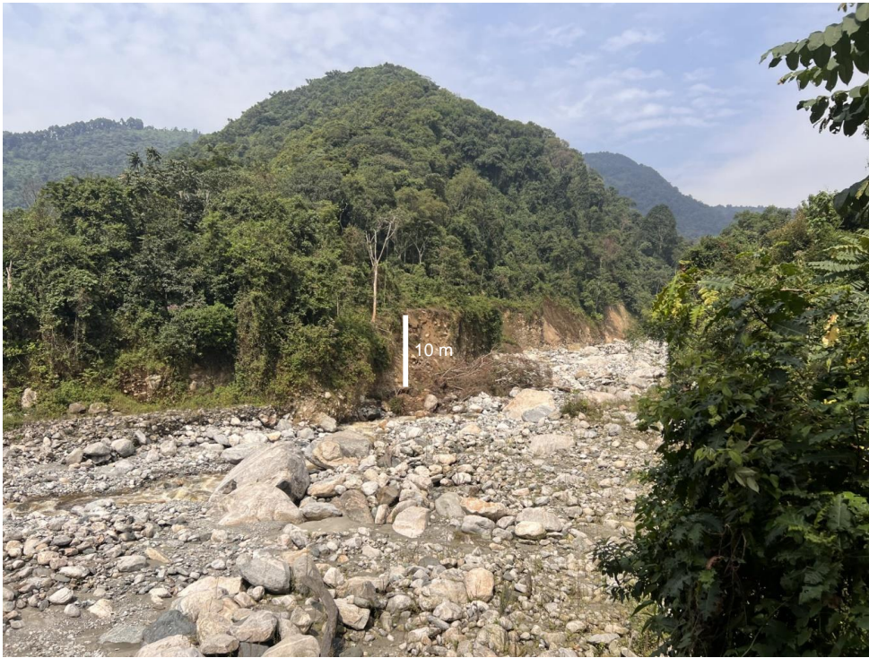
922 923 Figure I2: Landslide scar at 0.23758N, 29.97570E – 1 August 2024. 924 925 926 927 928 929 930 931 932
