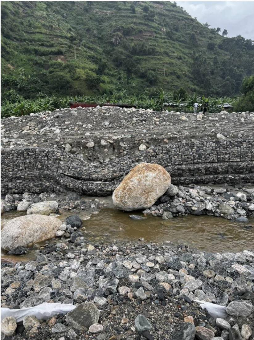
Figure H2: 0.21387N, 30.00558E, 7 June 2023 (damaged gabions).
