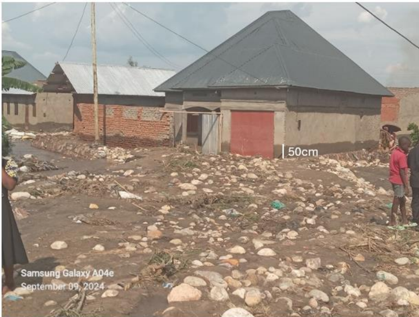
946 947 Figure L1: Photograph following flooding in Kasese town evidencing the inundation level and post-flood ground 948 contamination. Photograph provided by the Ministry of Water and Environment.
