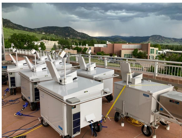
Figure 2: The 7 ASSISTS on the top of the NOAA building in Boulder, CO. The ASSIST-07 has a slightly different enclosure than the others, and is seen on the righthand side of the image. Photo by Laura Bianco.
