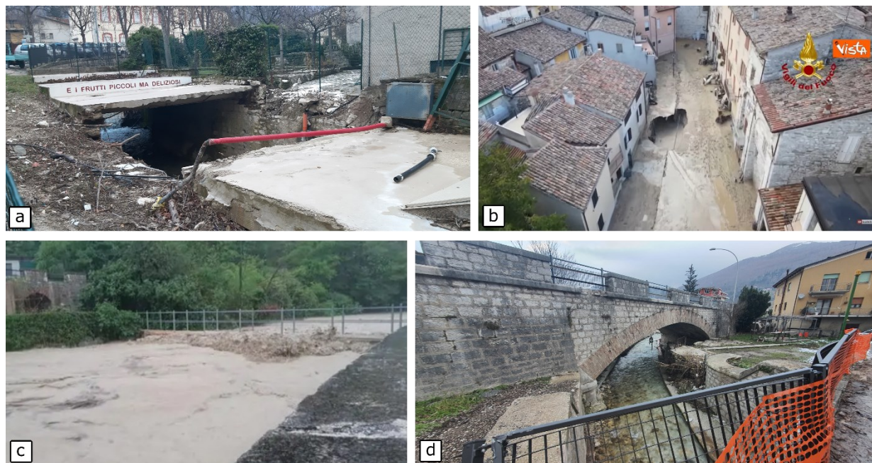
Figure 25: a) collapse of the tombed sections in Tumiat Street, Tenetra Creek; b) explosion of the buried sections in Fiorucci Street, Bevano Creek (courtesy of National Fire Department); c) undersized footbridge reached by the water level, subsequently washed away, Burano River; d) narrowing of bridge arch partially occluded by sediment and anthropogenic material, Bevano Creek.
