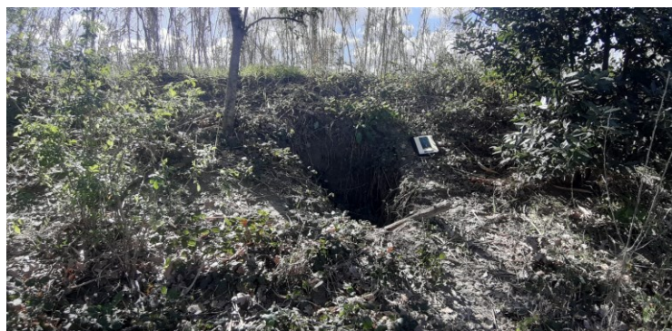
Figure 37: The burrow of fossorial animals along the right embankment of Misa River in the hamlet of Borgo Catena (Senigallia), with A4 block notes for scale.
