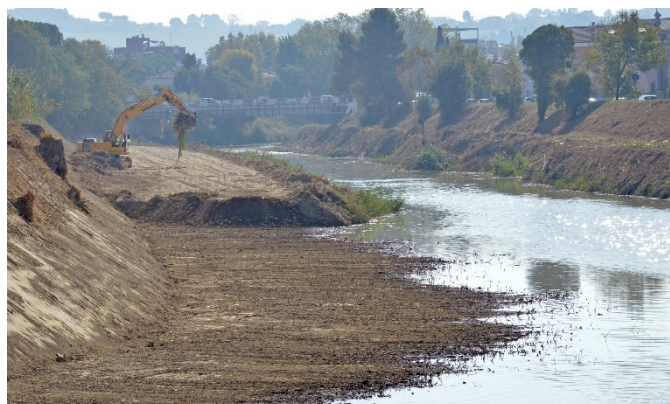
Figure 40: The works for the removal of river point bar sediments along the Misa River in Senigallia were executed in 2023. Image from https://www.adriaeco.eu/2023/10/13/alluvione-2022-sopralluogo-a-senigallia-per-la-verifica-dello-stato-dei-lavori-sul-misa/ (accessed on 12.16.2024).
