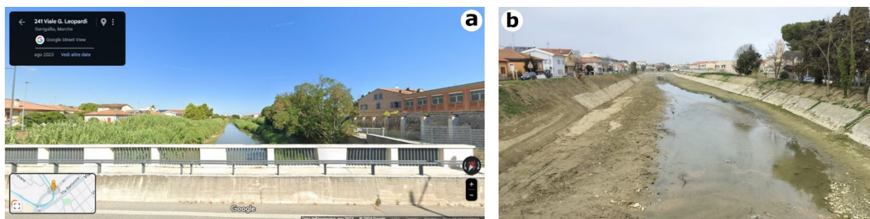
Figure 39: Two images of the same stretch of Misa River caught from Portone Bridge along Leopardi Street: a) in August 2023 (Google Earth image); b) in February 2024, after the works of the hydraulic section widening with the removal of sediments and vegetation.
