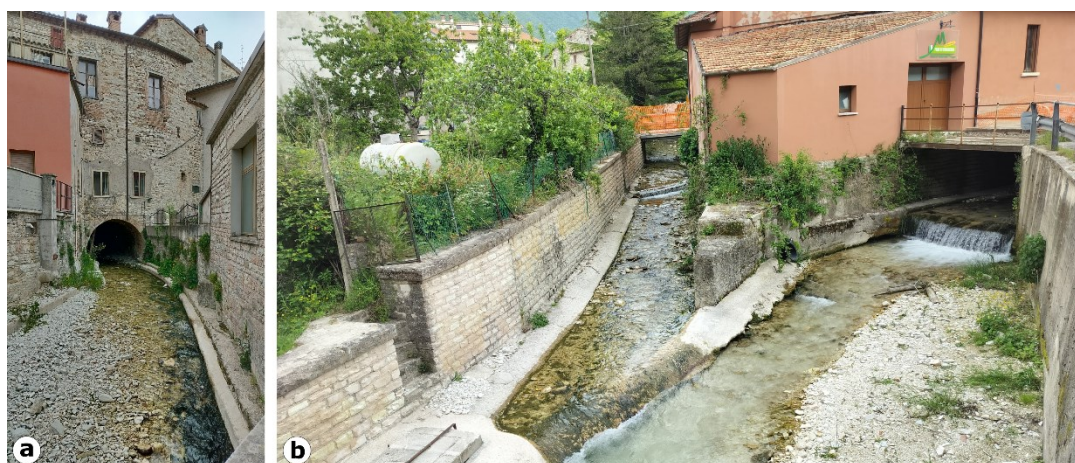
Figure 21: a) the Tenetra ditch channelled below a dwelling in the historical centre of Cantiano; b) the confluence between Tenetra (left) and Bevano creeks (right) in the historical centre of Cantiano with the channelled watercourses.
