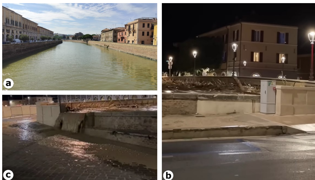
Figure 38: Three situations close to the 2 June bridge: a) the masonry embankments of Misa River in Senigallia seen from the 2 June bridge after heavy rain; b) the 2 June bridge with the intrados occluded by vegetation carried by the river a few moments (11:30 p.m. of 15 September 2022, Italian time) before the flood (youtube page of Storm Chasers Marche); c) the precise moment (00:05
