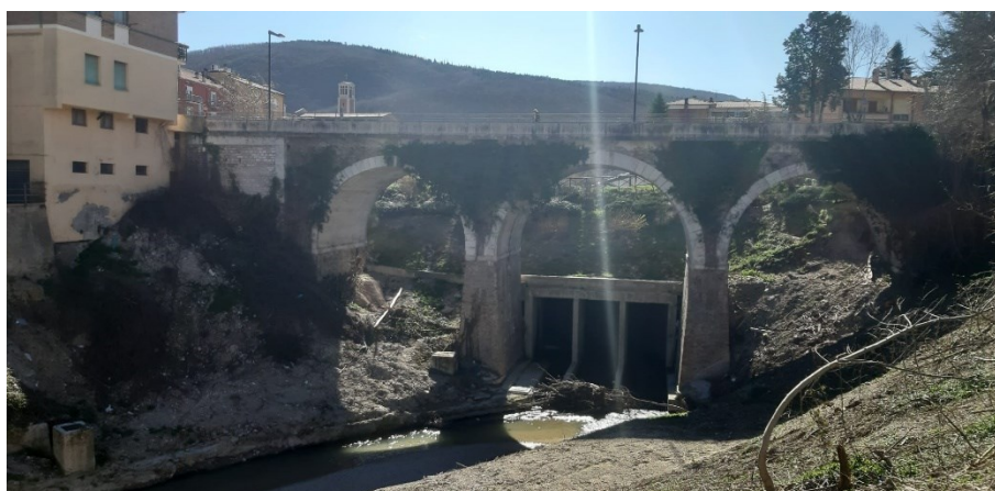
Figure 29: The Garibaldi Street Bridge saw from upstream with the evident, extreme reduction of the original flow section with a box-like structure (the markers on the wall on the left mark the hydrometric levels reached).
