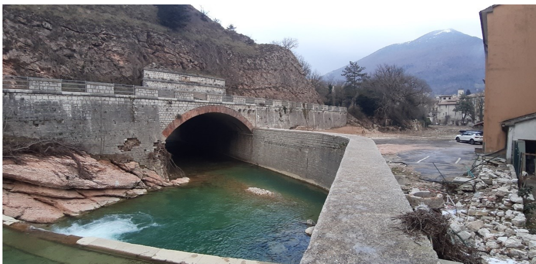
Figure 22: The 65-meter tunnelling of the Burano River below the calcareous mountain ridge, with the anthropogenic embankment behind which the alluvial plain, the parking and the historical centre are recognizable.
