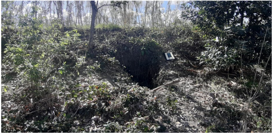
Figure 24: The burrow of fossorial animals along the right embankment of Misa River in the hamlet of Borgo Catena (Senigallia), with A4 block notes for scale.
