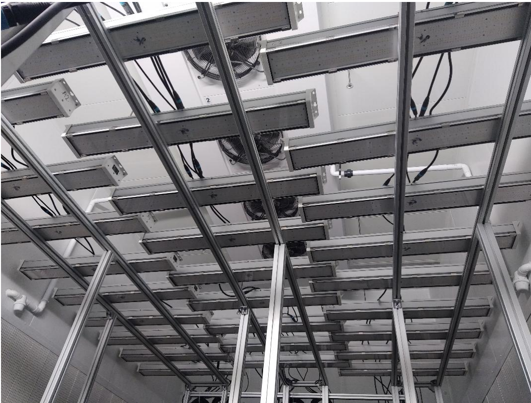
Figure 1: Photograph of the chamber's ceiling
