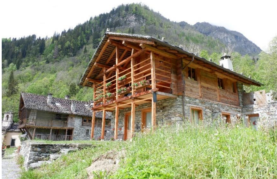
Figure 65 65 : Typical Walser house, an example of vernacular architecture in Alagna Valsesia. Photo by the authors
