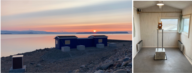
40 Figure 1: The Arctic magnetic observatory at Pituffik, with IAGA code PIF. Left: Exterior view of the observatory. The variometer enclosure is visible in the far-left corner, with the absolute building in the centre connected via a corridor to the electronics building on the right. Right: Interior of the absolute building, showing the fluxgate theodolite mounted on Pillar A (centre) and the scalar instrument located in the upper left corner on location F .
