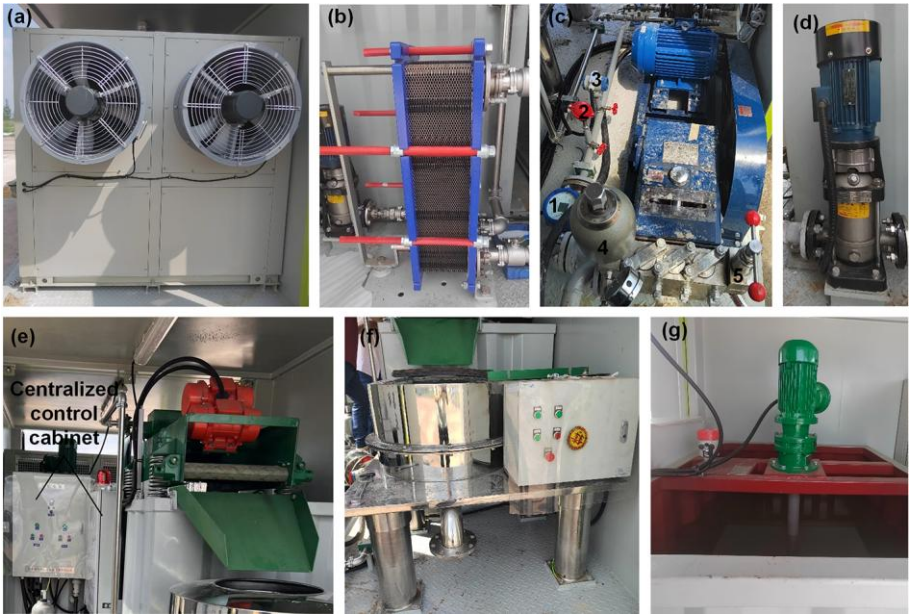
Figure 106: Main components of the DFCS: (a) refrigerating machine; (b) heat exchanger; (c) drilling-fluid pump; (d) vibration sieve; (e) vertical centrifuge; (f) circulating pump; and (g) stirrer.
