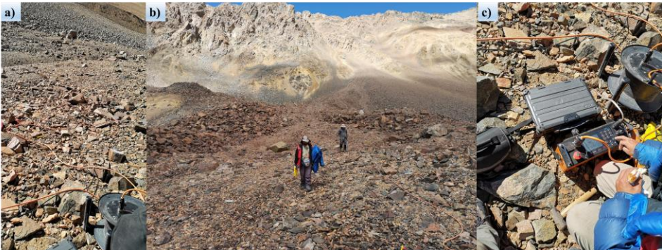
353 354 Figure 6. Photography of the fieldwork rock-glacier surface. (a) Intelligent multi-electrode cable reel used for deploying the ERT 355 array across the periglacial terrain. (b) Installation of the 600-m geoelectric line. (c) Operation of the ARES II resistivity meter 356 during data acquisition.
