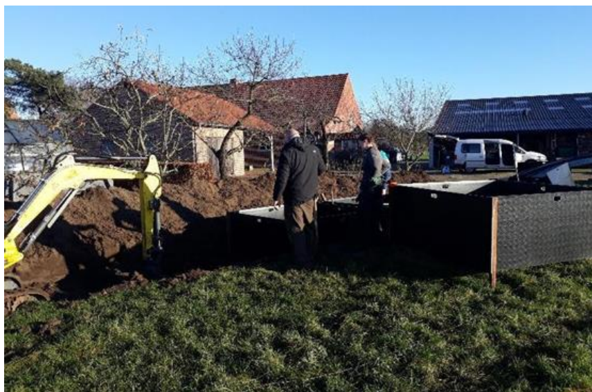
Figure A5. Excavation works during set up of experimental site, showing the black impermeable plastic boxes and the crane used for de-compaction
