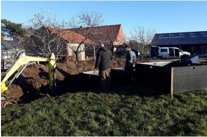
Figure ASA 6 . Excavation works during set up of experimental site, showing the black impermeable plastic boxes and the crane used for de-compaction
