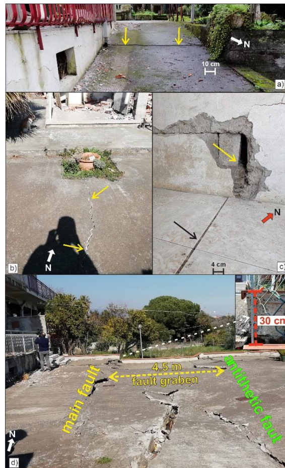
Figure 5: 26 December 2018 coseismic ruptures at Fiandaca trench site (see photos location in Fig. 4): a) ground rupture along a private road with few cm of offset; b) ground rupture which follows a damaged building wall, offset ~1 cm; c) 1.5 cm horizontal offset between two floor tiles continuing into the wall; d) fault graben on a private asphalt parking which extends over the wall and farmland. Photos taken on: 26 th December 2018 (a); 22 nd January 2019 (b and c); 18 th February 2019 (d).
