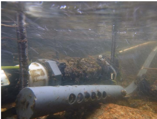
560 Figure 3: Pictures of the strainers and baffles in the station of Naizin (top) and Strengbach (bottom) to prevent clogging of the pumps.
