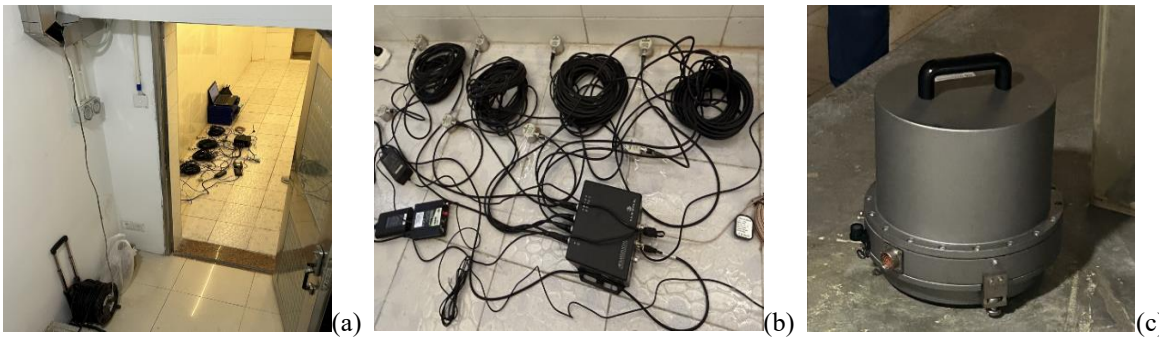
Figure 5: Set-up of monitoring system.(a) Interior view of tunnel; (b) AE acquisition device; (c) Seismometer.
