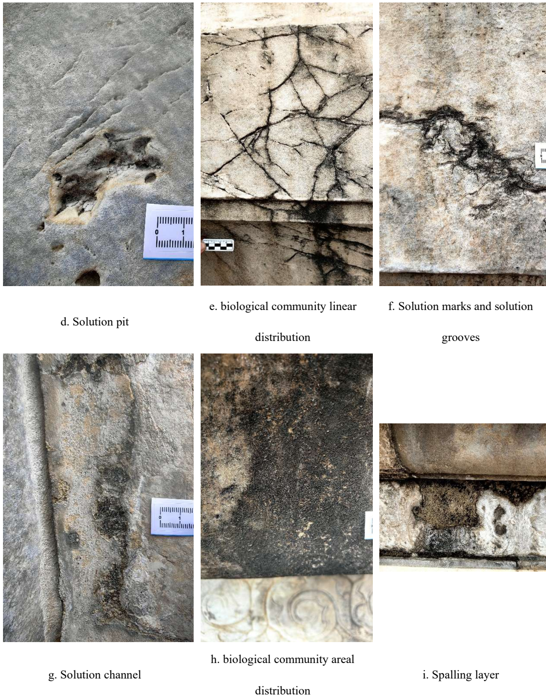
Fig. 22 Bioweathering forms on the marble surface of the Altar of Prayer for Good Harvests in the Temple of Heaven, Beijing, China.
