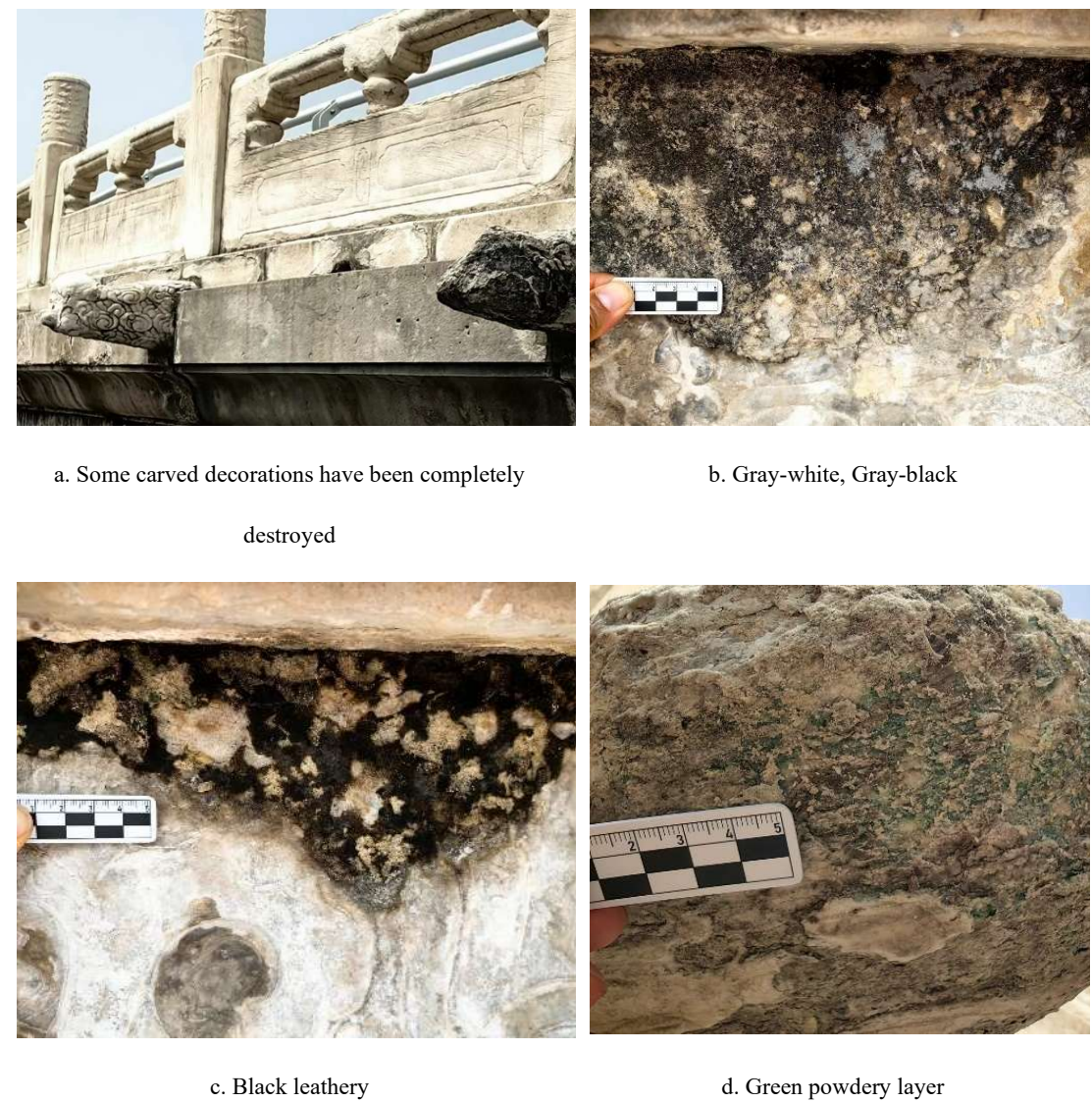
Fig. 13. Field photo of biomes on the south facing marble surface of the altar of Prayer for Good Harvest in the Temple of Heaven, Beijing, China.
