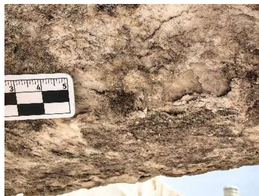
e. A loose, powdery layer has formed on the surface of the cloud chi heads, with a large amount of cyanobacteria growing inside.
