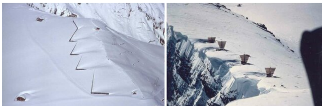
Figure. Snow fences to the left and wind baffles to the right in use in Switzerland (photos: Stefan Margreth).
