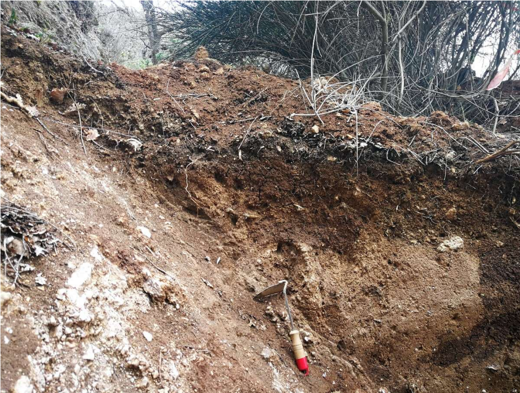
Figure S6. Southern wall of the trench TC. Detail of the bedrock fault plane.
