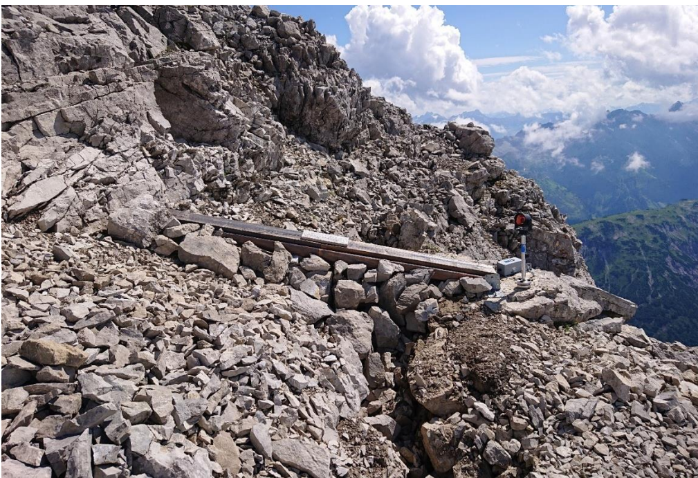
5 Fig. S 2: Photo of vibrating wire crackmeter "Crack06" with wood roof.
