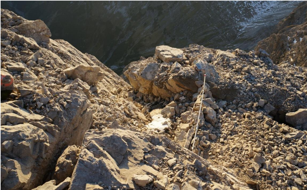
Fig. S 1: Photo of vibrating wire crackmeter "Crack06" without its protective wood roof.
