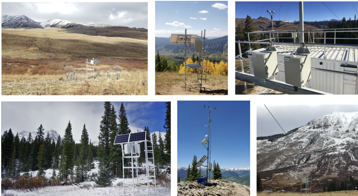
Figure 2. Photos of the six sites in SAIL-Net. From left to right, top to bottom, the sites are Pumphouse, Snodgrass CBMid, Irwin, CBTop, and Gothic. Four of the sites ran on solar power, and the solar panels can be seen in the photos. CBMid and Gothic both ran on ground power.
