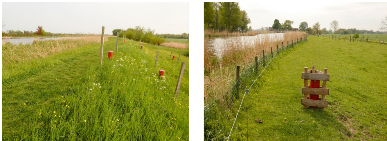
60 Figure 1 Two examples of canal dikes in the Netherlands: Duifpolder polder is shown at the left and the Drooggemaakte Geer- en Kleine Blankaardpolder is depicted at the right. In both images, the canal has permanent high water levels close to the crest level (on the left side) and the low-lying polder is mainly used for agriculture (on the right side). The head difference between the canal water level and water level in the polder are 2.7m (Duifpolder) and 4.3m (Drooggemaakte Geer- en Kleine Blankaardpolder). The red tubes protect the measuring equipment and the piezometers used to measure the hydraulic head. Photos by EURECO/Cyril Liebrand, 2022.
