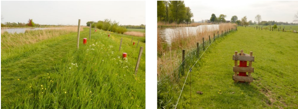
Figure 1 Two examples of canal dikes in the Netherlands: Duifpolder is shown at the left and the Drooggemaakte Geer- en Kleine Blankaardpolder is depicted at the right. In both images, the canal has permanent high water levels close to the crest level (on the left side) and the low-lying polder is mainly used for agriculture (on the right side). The head differences between the canal water levels and water levels in the polders are 2.7m (Duifpolder) and 4.3m (Drooggemaakte Geer- en Kleine Blankaardpolder). The red tubes protect the measuring equipment and the piezometers used to measure the hydraulic head. Photos by EURECO/Cyril Liebrand, 2022.
