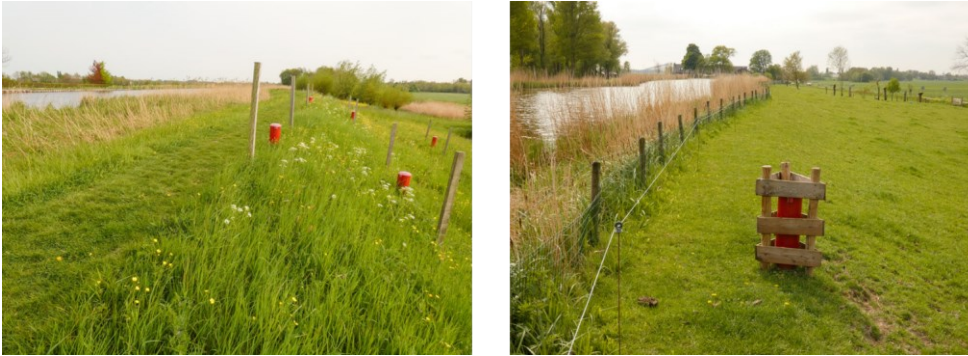
Figure 1 Two examples of canal dikes in the Netherlands: Duifpolder polder is shown at the left and the Drooggemaakte Geer- en Kleine Blankaardpolder is depicted at the right. In both images, the canal has permanent high water levels close to the crest level (on the left side) and the low-lying polder is mainly used for agriculture (on the right side). The head differences between the canal water levels and water levels in the polders are 2.7m (Duifpolder) and 4.3m (Drooggemaakte Geer- en Kleine Blankaardpolder). The red tubes protect the measuring equipment and the piezometers used to measure the hydraulic head. Photos by EURECO/Cyriel Liebrand, 2022.
