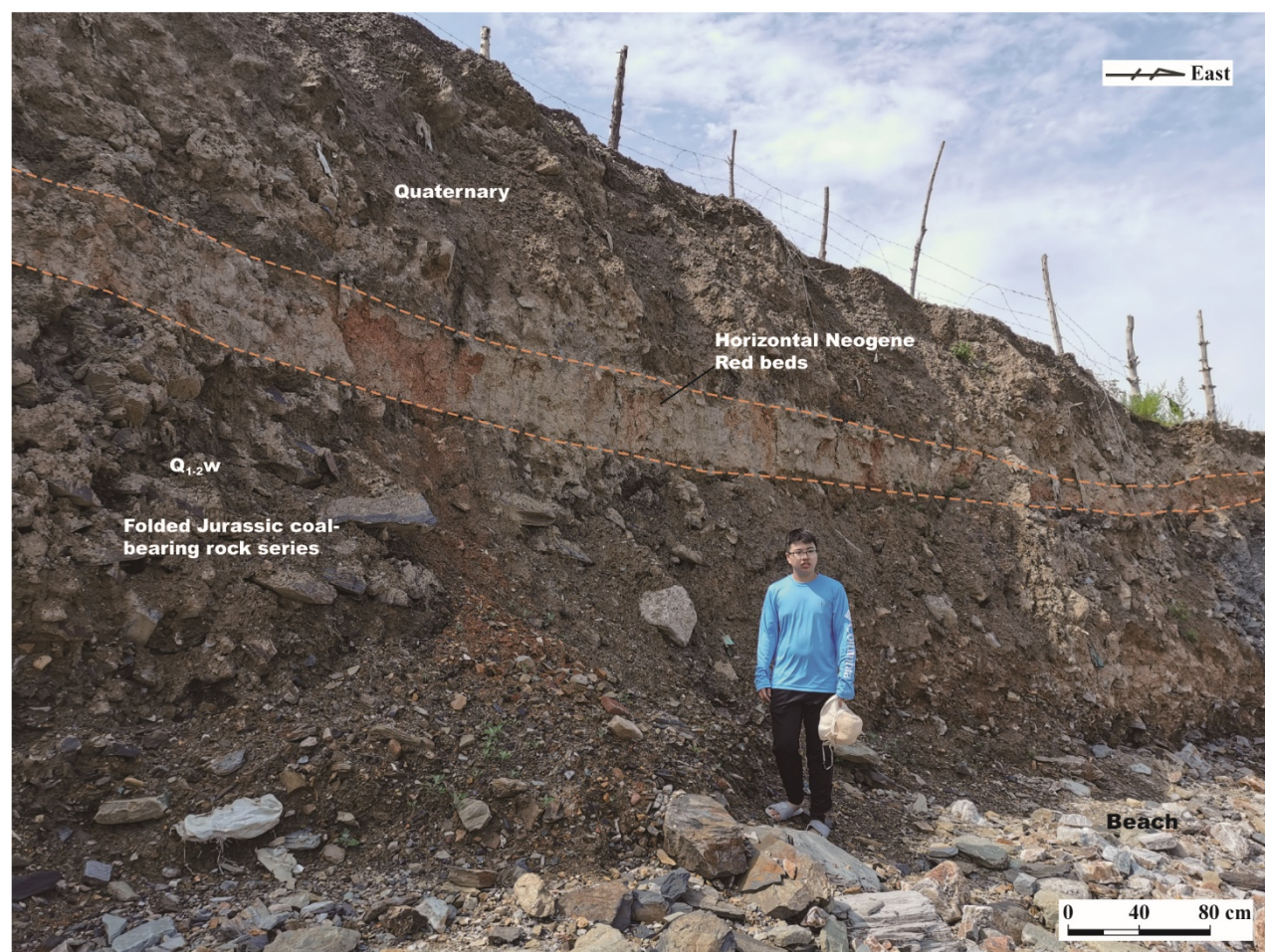
Figure 8: Coastal cliff occurs at the southernmost edge in eastern coast of the Liaodong Peninsula, showing the vertical cutting of the horizontal Neogene red bed due to active normal faulting. Q 1-2w , Lower-Middle Jurassic Wafangdian Formation.
