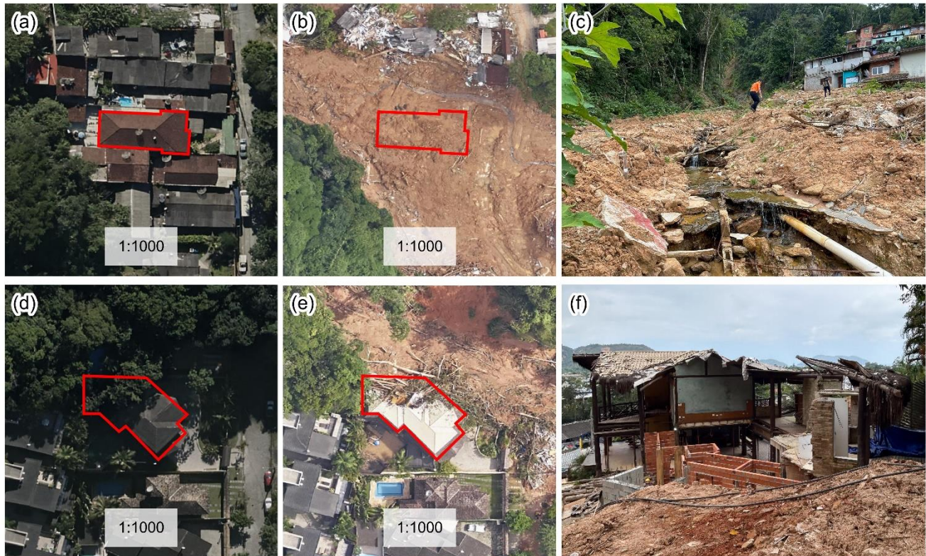
165 Figure 2. Examples of total destruction and partial damage to buildings. (a) Pre-disaster aerial view of a building that was totally destroyed; (b) Post-disaster aerial view of the total destruction to the building (a); (c) Photograph from a field visit at the site where the building (a) was located, taken in November 2023; (d) Pre-disaster aerial view of a building that was partially damaged; (e) Post-disaster aerial view of the partial damage to the building (d); (f) Photograph from a field visit of the remnants of the building (d), taken in November 2023. Data source: Aerial imagery from DataGEO (2023).
