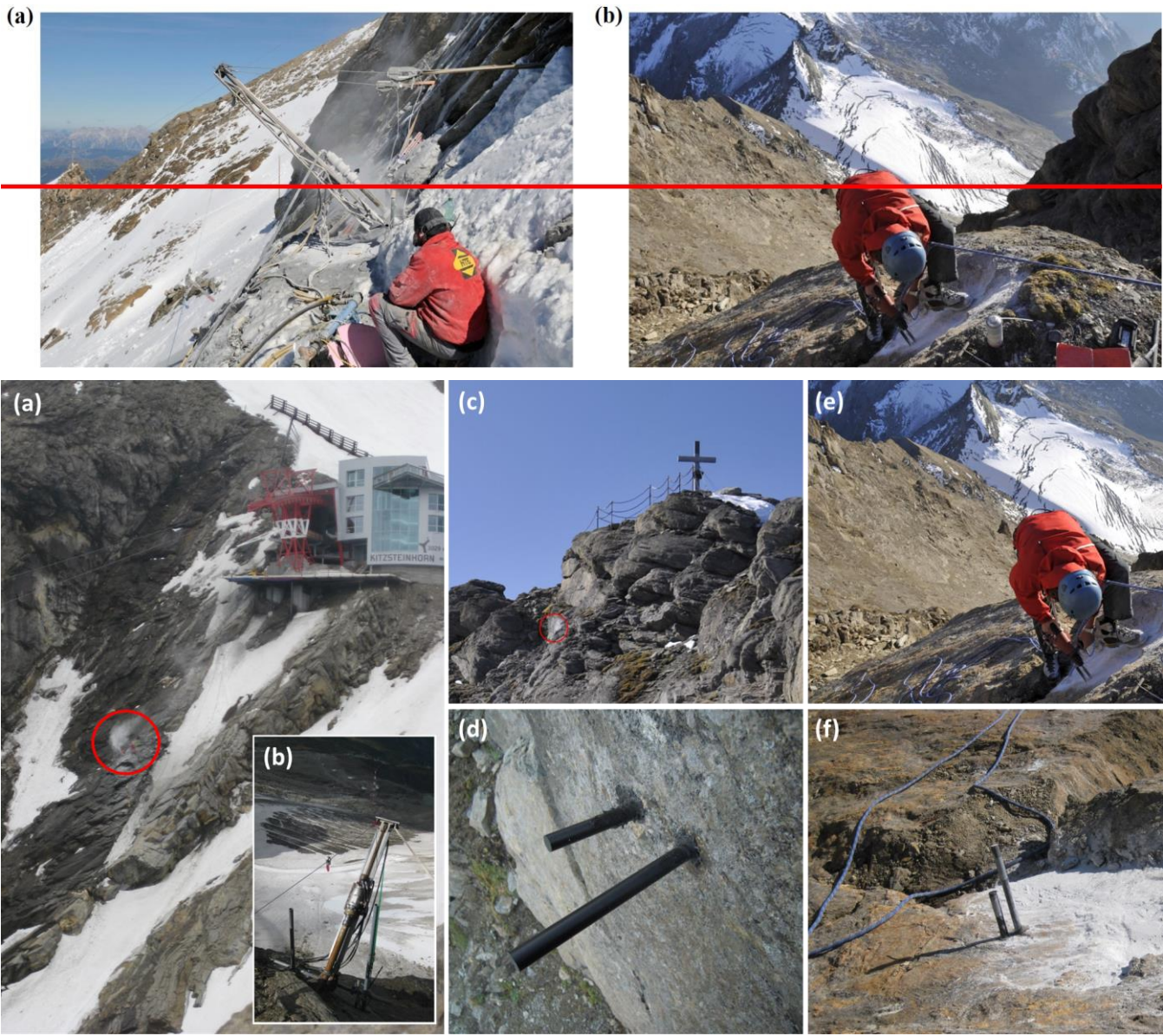
Figure 2: (a) Drilling works at DB in the Kitzsteinhorn north-face (07.07.2011); (b) Drilling equipment at DB (17.08.2011); (c) Location of SB 3 below the Kitzsteinhorn summit (06.10.2011); (d) Close-up of SB 3 (31.07.2013); (e) Drilling works at SB 4 (05.10.2011); (f) Close-up of SB 4 (05.10.2011) (all photos taken by I. Hartmeyer). (a) Drilling procedure (air-flushed rotary drilling) for a 30 m deep borehole (DB) on the western flank of the Kitzsteinhorn (Austria) (identical procedure to the DB used in this study); (b) Drilling of a shallow borehole (SB) for the installation of Ibuttons® for temperature logging at a depth of 0.1 m on the southern flank of the Kitzsteinhorn (2011). Due to the lower effort, more measuring points could be realized to address spatial variability. Photos by Ingo Hartmeyer.
