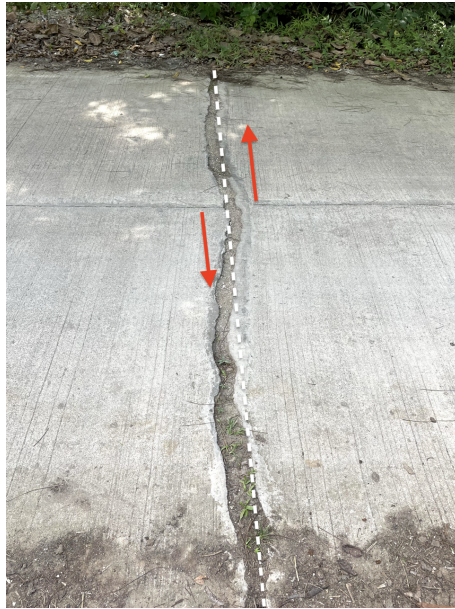
Figure S8: Pt FP5. Ruptured road section showing sinistral offset and perpendicular separation. Point is visible in OIC.
