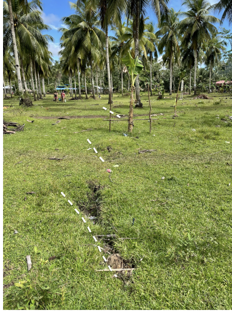
Figure S10: Pt FC5. Right stepping en echelon fissures along the fault trace near the unfinished house.
